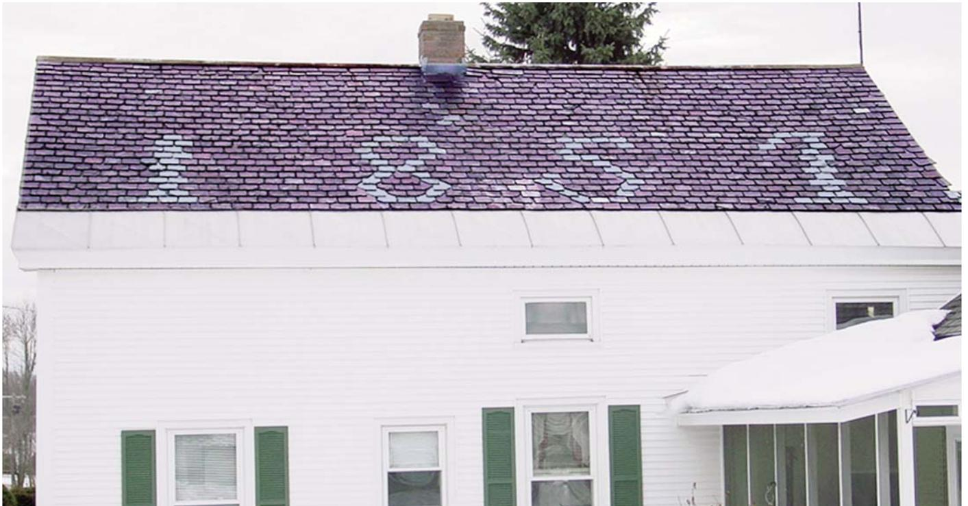
*This 150-year-old roof was built of Vermont slate on wood decking and probably nailed with hot-dipped galvanized nails.*
