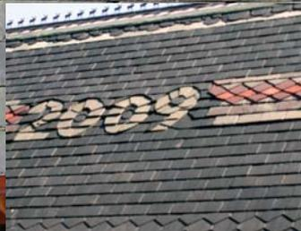
same methods explained above. All the black slate on this side is North Country black. I also used red, purple and green in the roof. Along with that, we designed and installed a different ornamental band with diamond shapes. At the bottom, I installed a simple octagonal pattern.
