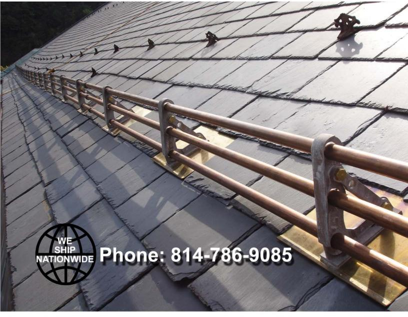
Snow guards, snow rails and snow fence made of copper, bronze, brass, aluminum and stainless steel, for asphalt, slate, tile and metal roofs, including flat metal and standing seam.
