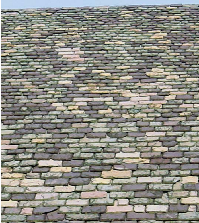
Figure 5: Graduated slate roof at Grove City College, Grove City, Pennsylvania. Slates vary in both widths and lengths. This roof also blends several colors of slate.
