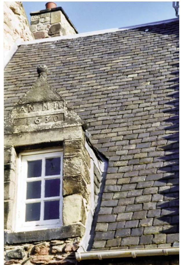
Traditional Scottish Slate Roof, Edinburgh, Scotland
